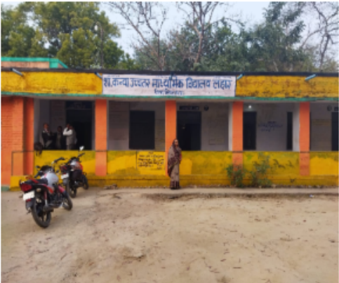
Polling Station Building Front View
