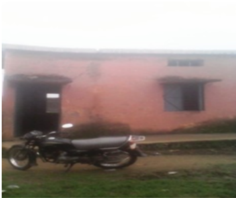
Polling Station Building Front View
