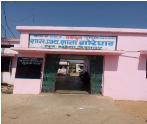
Polling Station Building Front View
