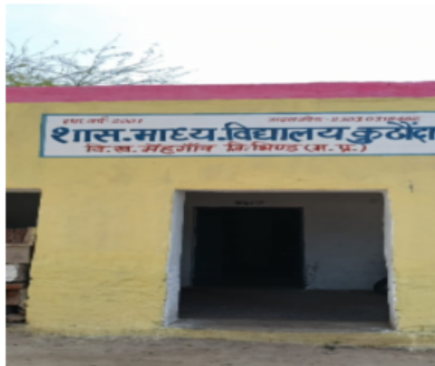
Polling Station Building Front View
