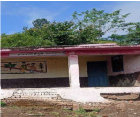
Polling Station Building Front View
