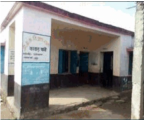
Polling Station Building Front View
