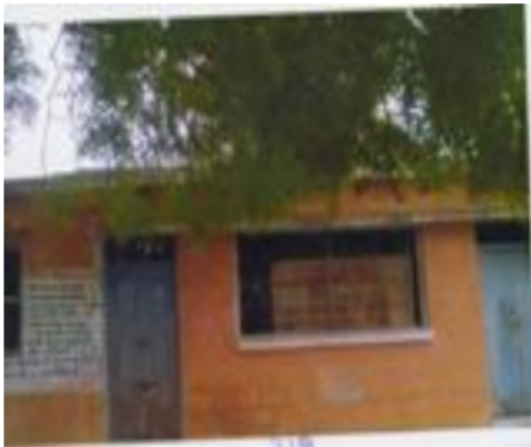
Polling Station Building Front View
