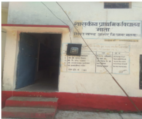
Polling Station Building Front View
