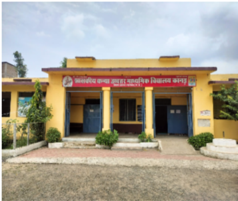
Polling Station Building Front View
