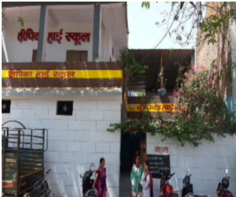
Polling Station Building Front View
