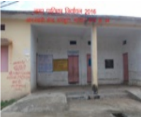
Polling Station Building Front View
