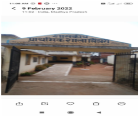
Polling Station Building Front View
