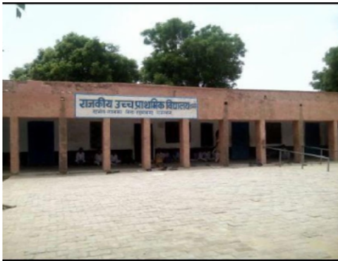
Building Front View
