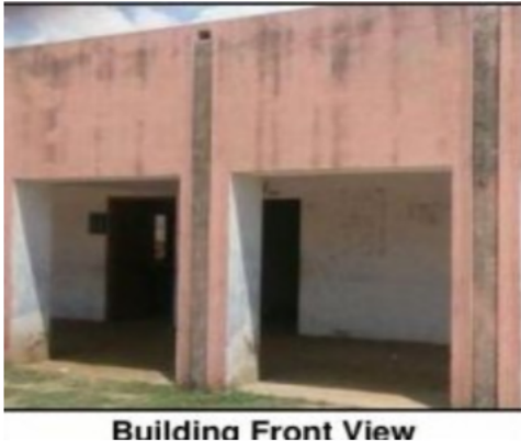
Building Front View
