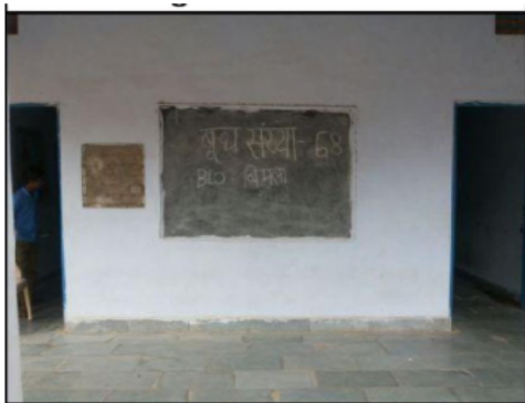
Building Front View
