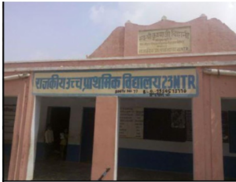
Building Front View
