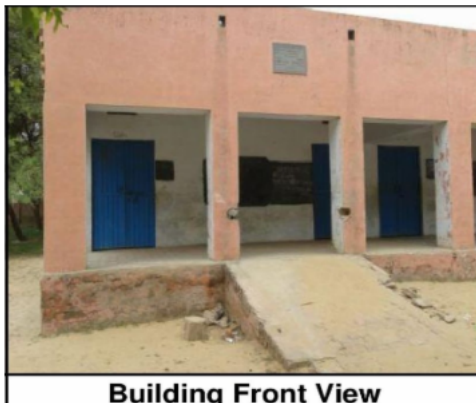
Building Front View
