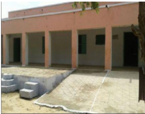
Building Front View
