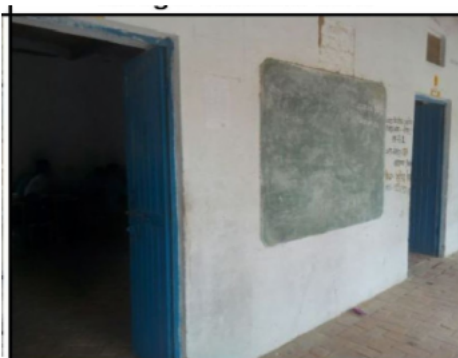
Building Front View
