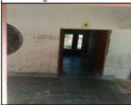
Building Front View
