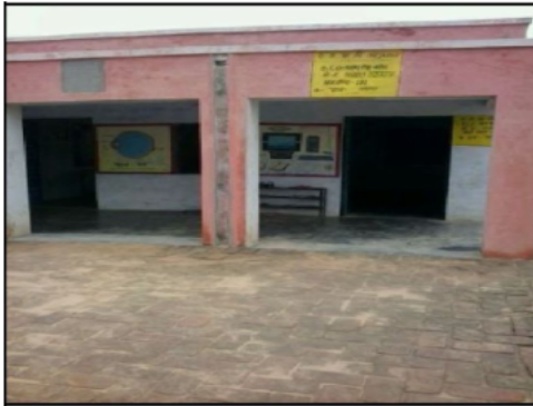
Building Front View
