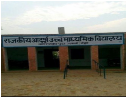
Building Front View
