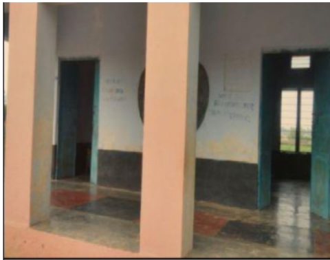
Building Front View
