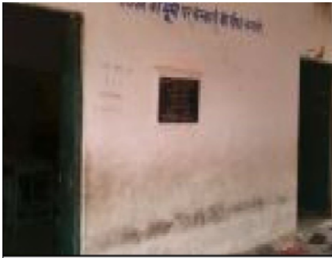
Building Front View
