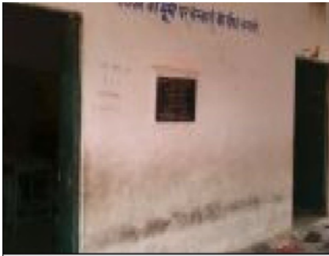
Building Front View
