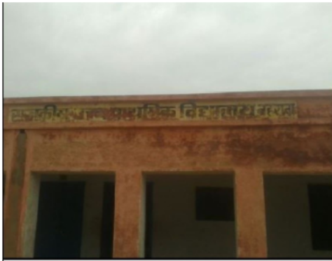
Building Front View
