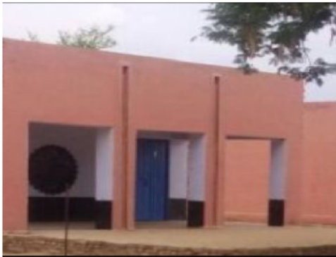
Building Front View
