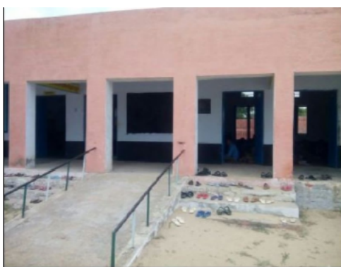
Building Front View
