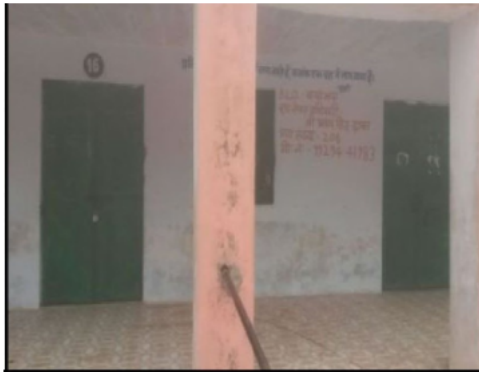
Building Front View
