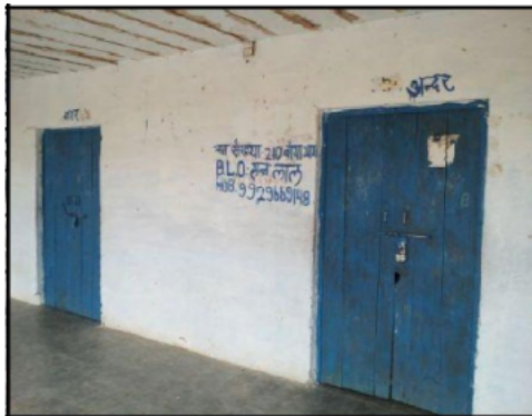
Building Front View
