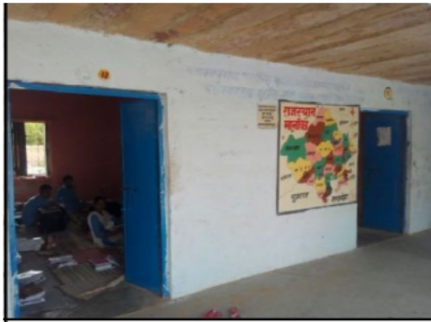
Building Front View
