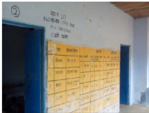
Building Front View
