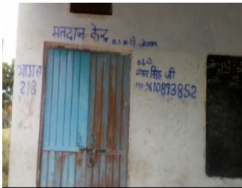
Building Front View
