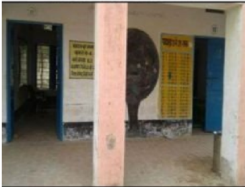
Building Front View
