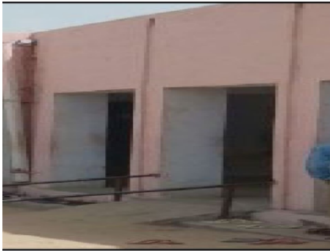
Building Front View
