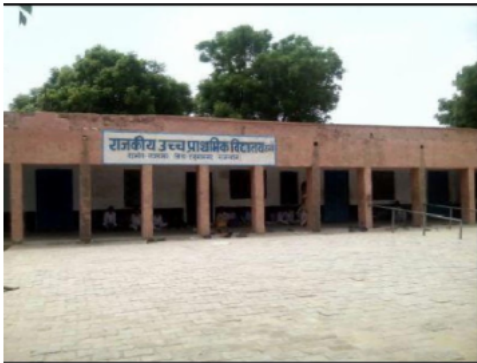
Building Front View
