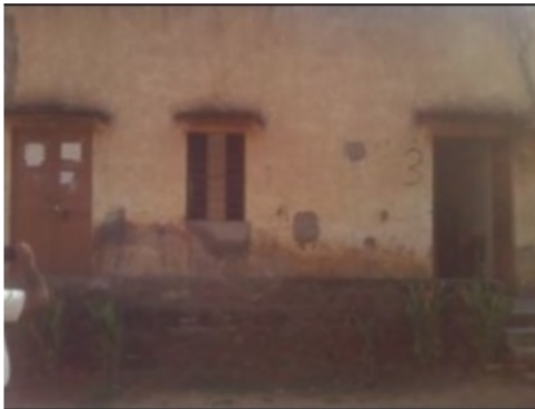
Building Front View
