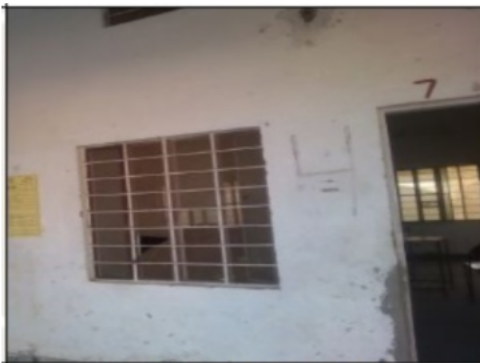
Building Front View
