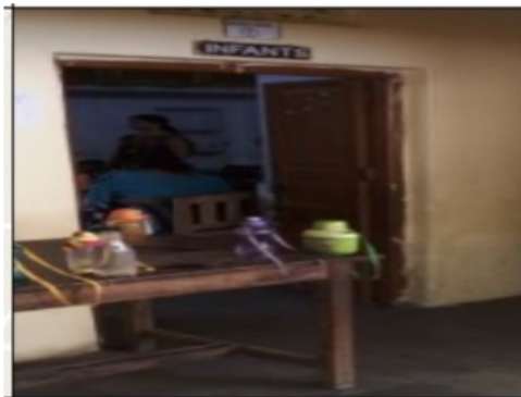
Building Front View
