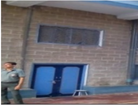
Building Front View
