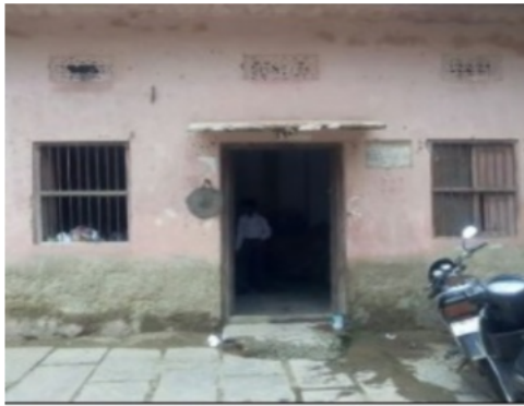
Building Front View
