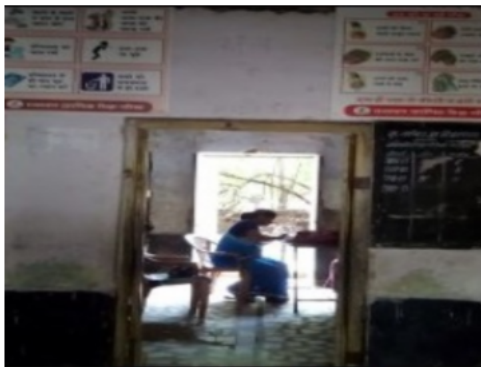
Building Front View
