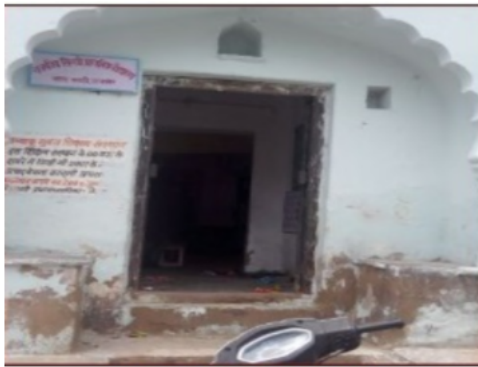
Building Front View
