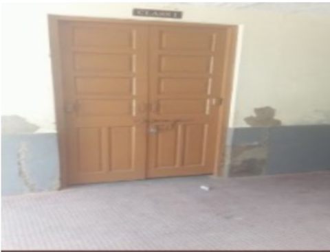
Building Front View
