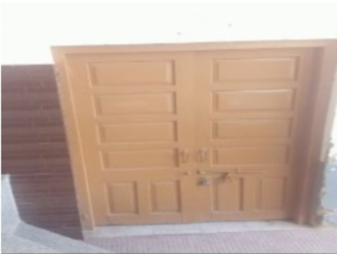
Building Front View
