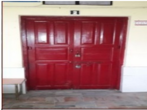
Building Front View
