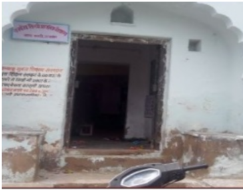
Building Front View
