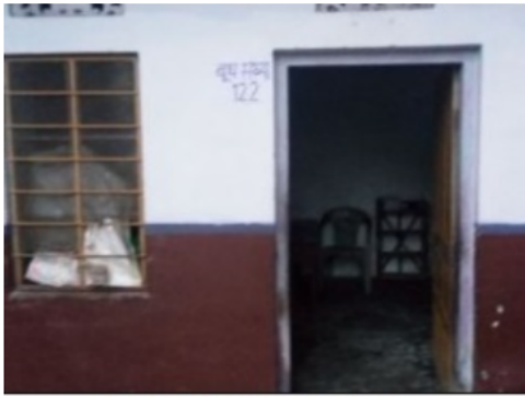
Building Front View
