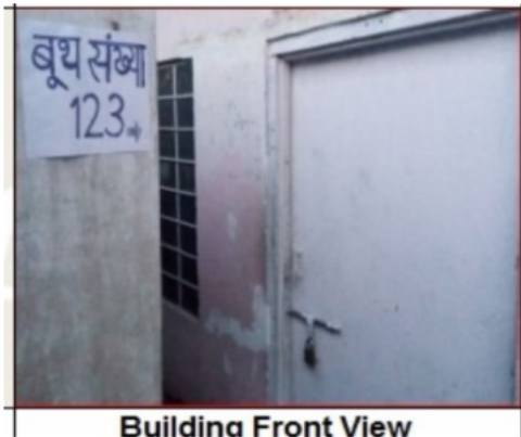
Building Front View
