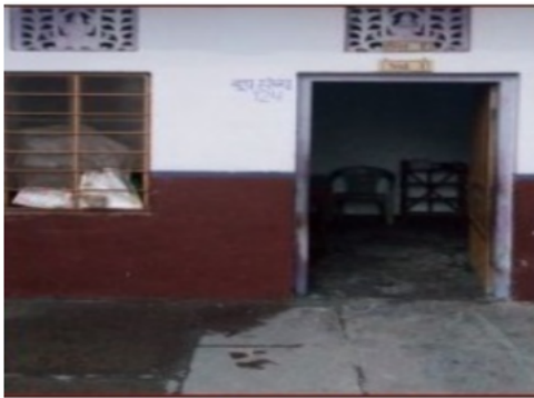
Building Front View
